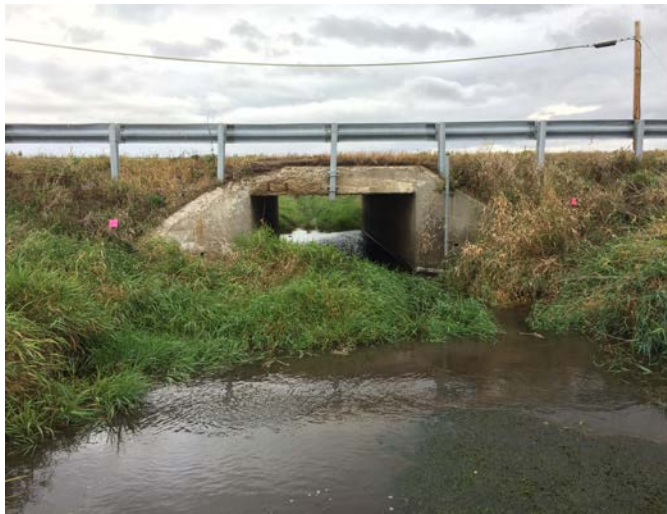
Photo 1: View of the west end of the Harmony Road over Harmony Creek culvert looking east.
