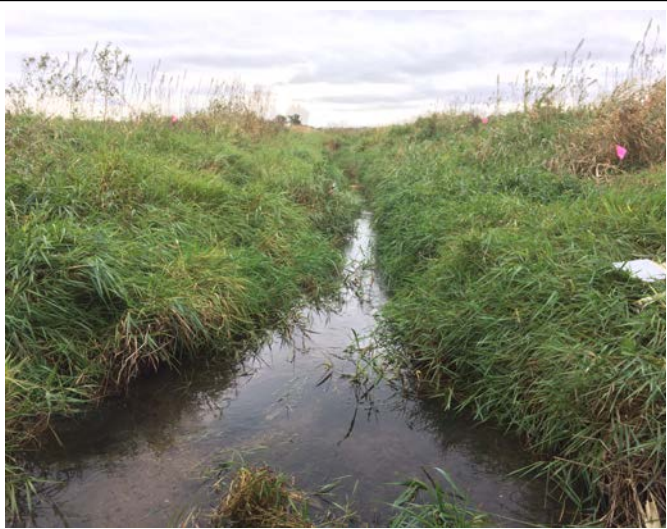
Photo 3: View from the culvert looking east upstream.
